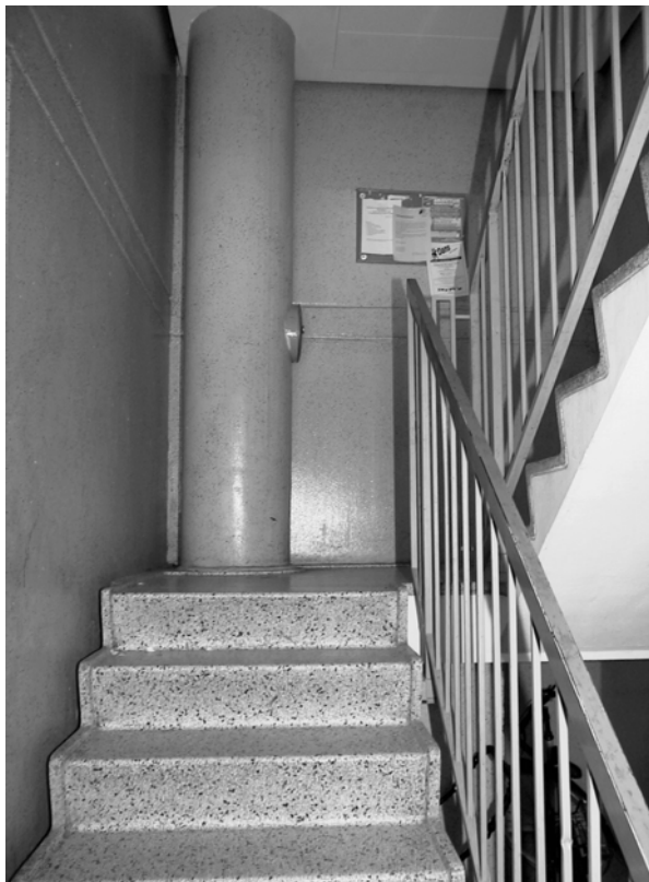
Figure 15. Indoor chute for the disposal of household refuse.
